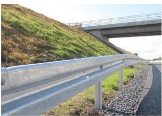
A. W Beam Crash Barrier: A typical guardrail system consists of a steel W-Beam rail on steel posts with various designs of end treatments and transitions made from the same material.
